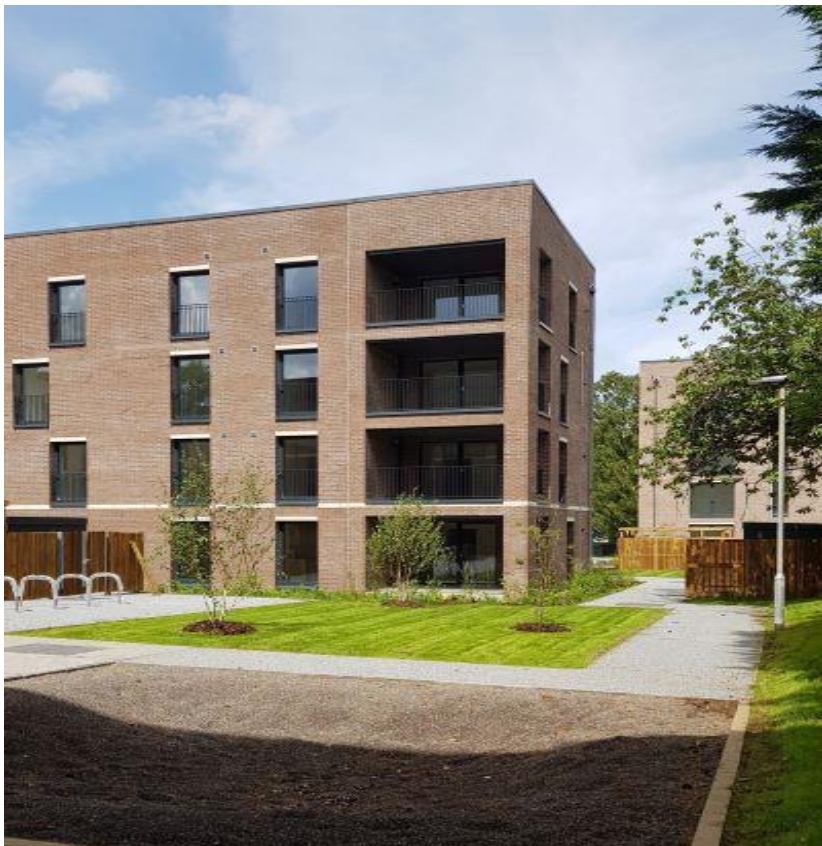
St. Andrew's Drive new build development
