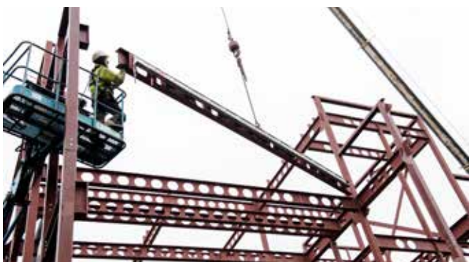
Work progressing at new homes in Pollokshields.
