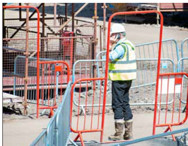
New homes at St. Andrews Drive, all of the tenants in Phase 2 of St Andrews were re-housed during the year and demolition will begin in August 2018.
