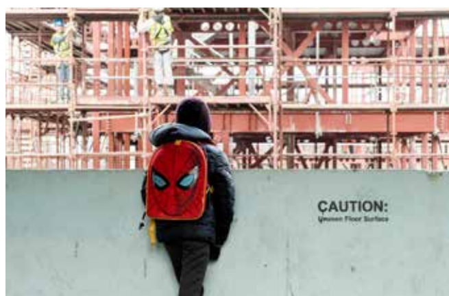
Spiderman checking out his new home from the remaining deck access flats, Pollokshields.
