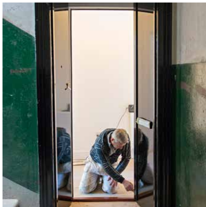
Private Acquisition Flats were refurbished at a cost £1.1m last year.
